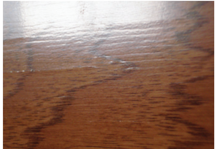
After a big relative humidity change, lathe marks in this rotary-peeled floor became apparent on the surface.
